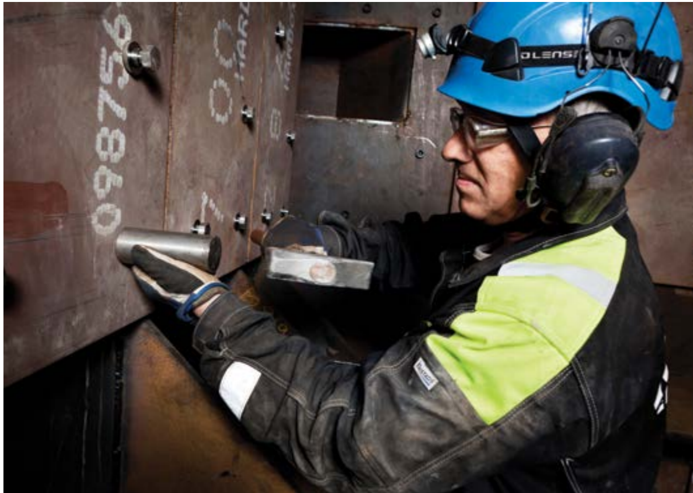
Installation of WRC socket screw.
